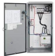
Enclosed soft starter, Controller 3RW44366BC34, Std. duty rating 50HP @230V, Std. duty current rating 145A Control voltage 115Vac Encl. type 4 painted steel, Water/dust tight for outdoors
