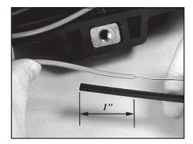
6.5 Snap the 3M<sup>™</sup> FibrTube into the intended splice tray entrance location. Cut the FibrTube near the end of the retainer slot.
