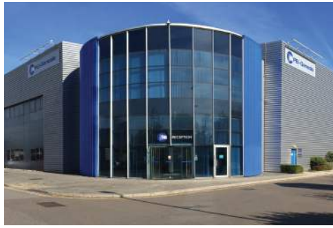
European Headquarters & Production Facility, Southampton, UK
