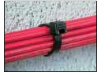
4. Install wires or cable.
