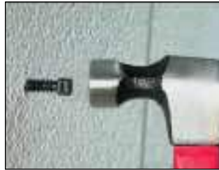
2. Hammer mount into hole.
