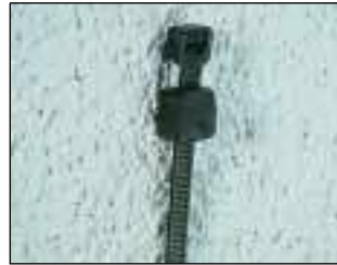
3. Place cable tie through mount.
