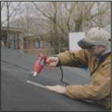
Weld Roofing Felt
