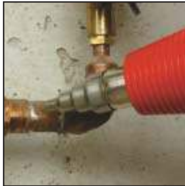
Solder Copper Pipe
