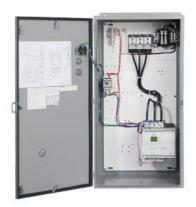
Enclosed soft starter, Controller 3RW44261BC34, Std. duty rating 50HP @460V, Std. duty current rating 68A Control voltage 115Vac Enclosure type NEMA 3/3R Weather proof outdoor use
