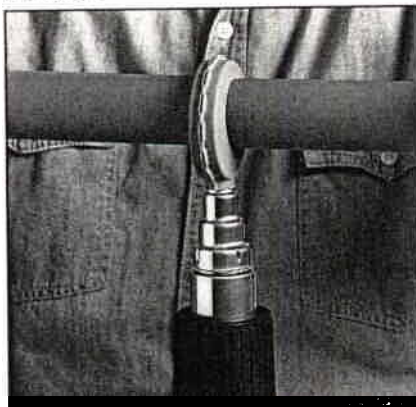
Welding with heat reflector
