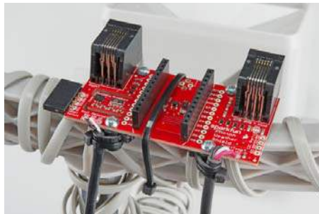
The snipped USB cable (right) and the DS18B20 cable (left), both secured to standoffs with zip ties.
