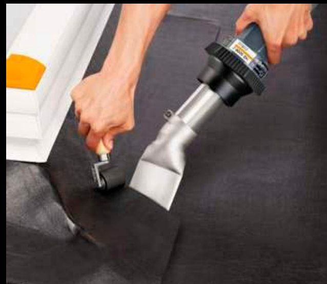
Overlap welding on a light dome.
