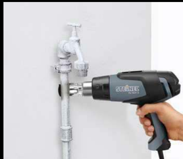
Thawing frozen pipes.
