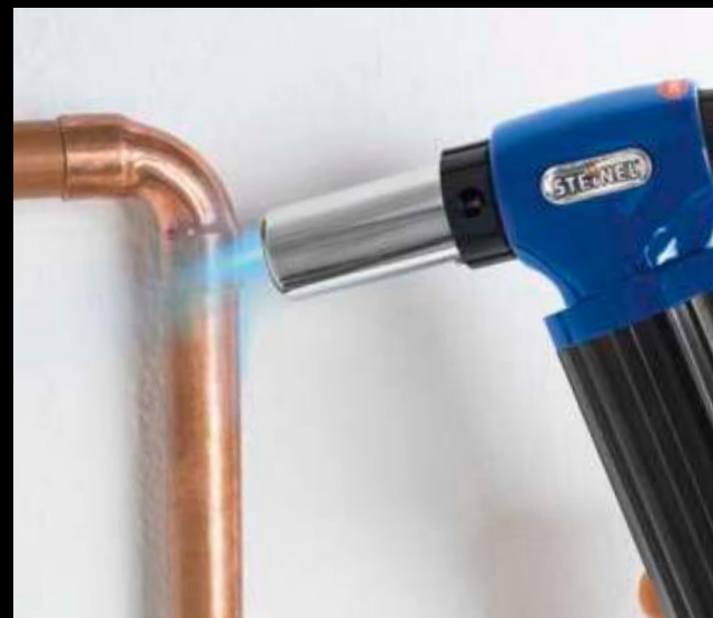
Solder joints on copper piping
