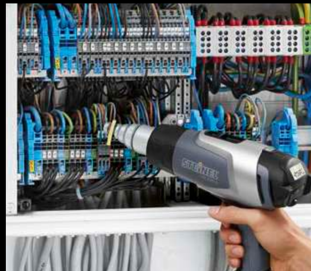
Shrinking cable sleeves in distribution cabinet
