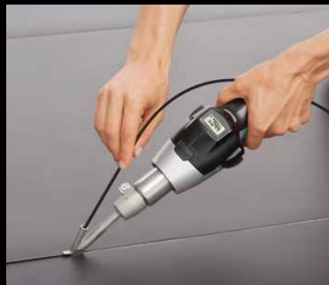
Welding linoleum floors.
