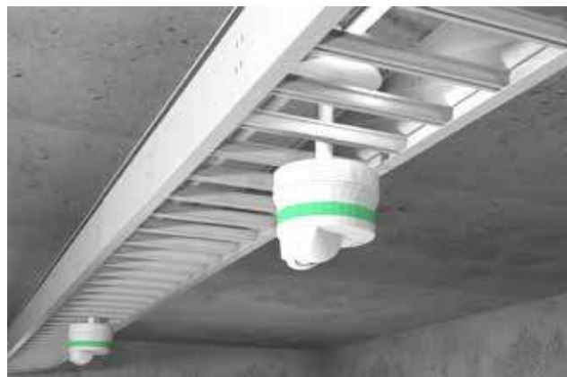
The sensor is placed outside the obstacle by using the SBPBASEA and a pipe
