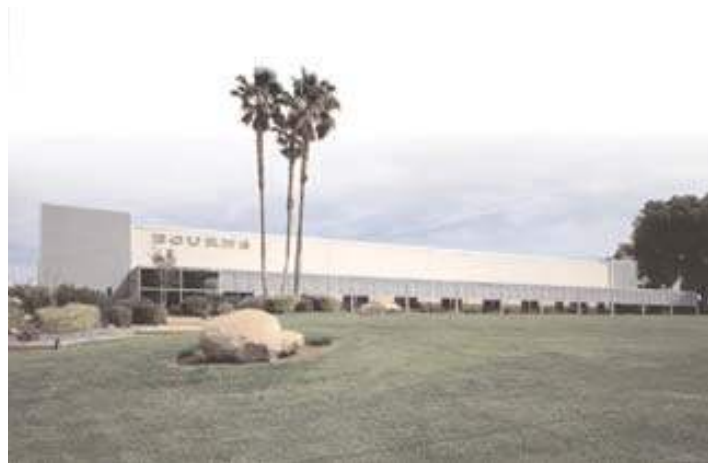
Bourns Corporate headquarters in Riverside, California
