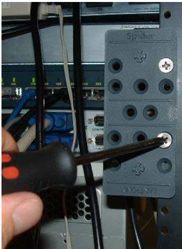
1. Mount the bracket with a Phillips-head screwdriver
