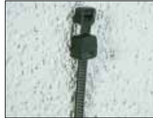
3. Place cable tie through mount.
