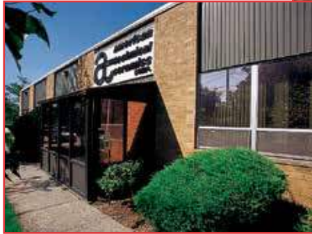
ATC's New York Facility occupies approximately 75,000 sq. ft.
