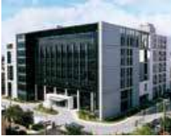
Taoyuan Technology Center (Green Building)
