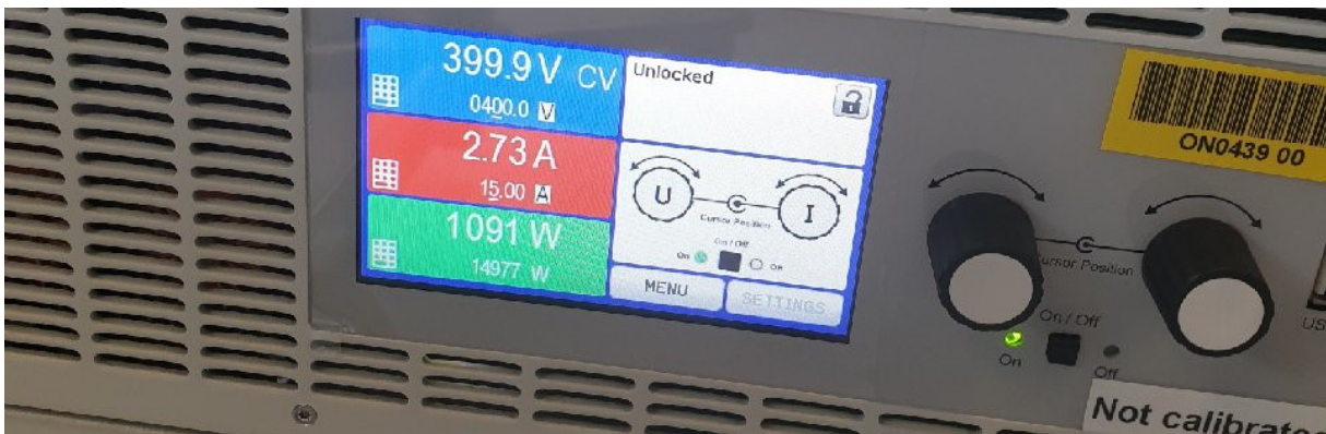
Figure 23. DC Power Supply Reading @ 1 kW.
