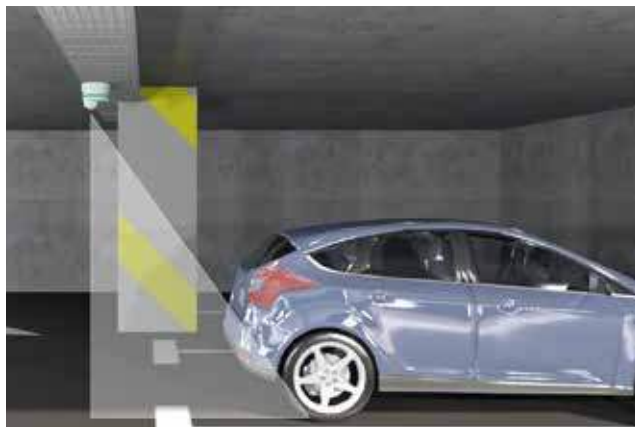
The sensor is wrongly mounted on the left hand of the cable tray
