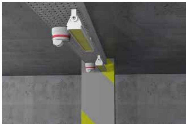
The LED lamp is wrongly mounted in front of the sensor
