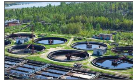
Water, wastewater treatment
