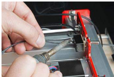
Soldering on the leads.
