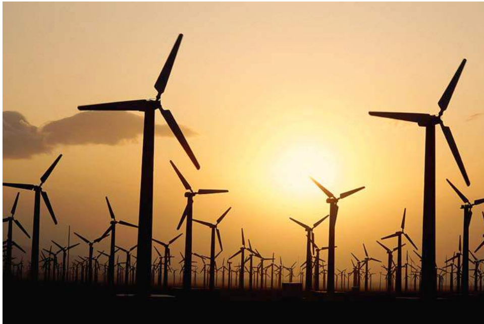
Photo 24. Fiber optics is used to transfer data at this wind-powered electric generating site because of low weight and noise-free transmission.
