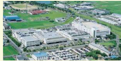
Solar Systems Group Electronic Components Group (Katsuragi, Nara Prefecture)
