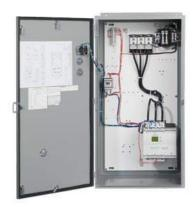
Enclosed soft starter, Controller 3RW44566BC35, Std. duty rating 750Hp @575V, Std. duty current rating 693A, Control voltage 115 AC, Non-combination type, Encl. type 4 painted steel, Water/dust tight for outdoors
