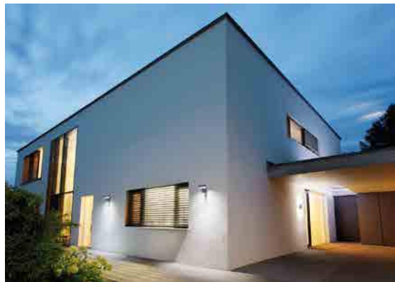
Residential outdoor lighting
